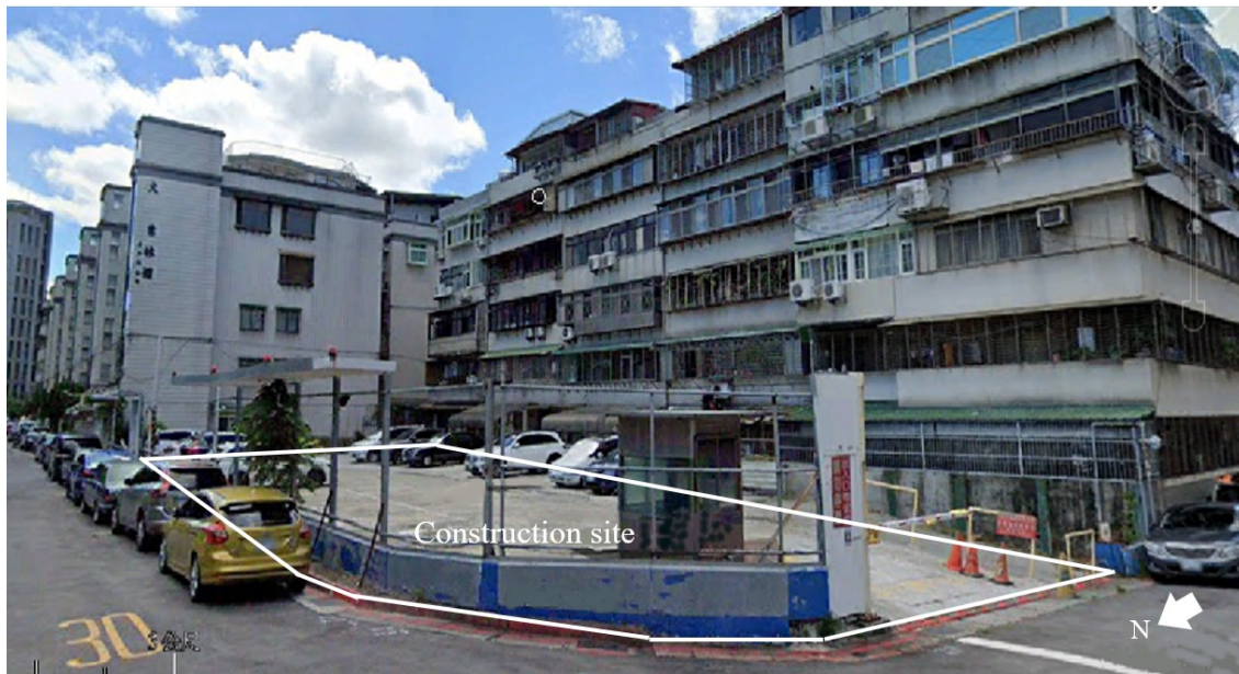
Figure 7. Construction site and adjacent roads and buildings before foundation excavation of the Jitai-Dazhi site (Taipei, Taiwan) (Google Earth, 2023).
