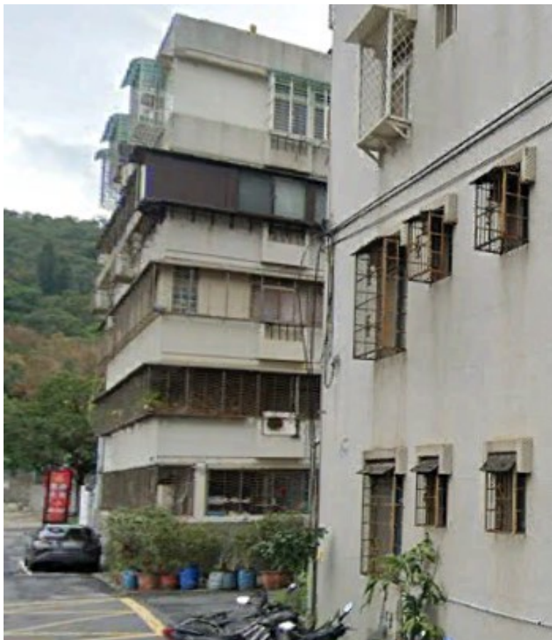
(a) Five stories before subsidence (Google Earth, 2023).
